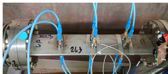
Figure 6: Vacuum pipe with different pickups (CBPM).
