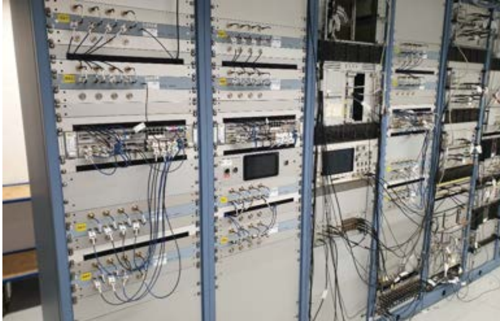
Three LiberAs (for twelve SIS18 BPMs) in Electronic room
