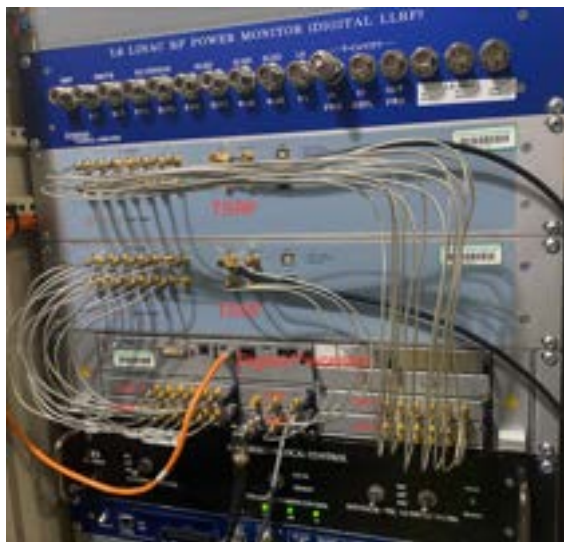
Figure 2: The first Libera LLRF system delivered to the APS. It consists of two TSRF units and one digital processor unit. Six AMC slots are marked in the photo.
