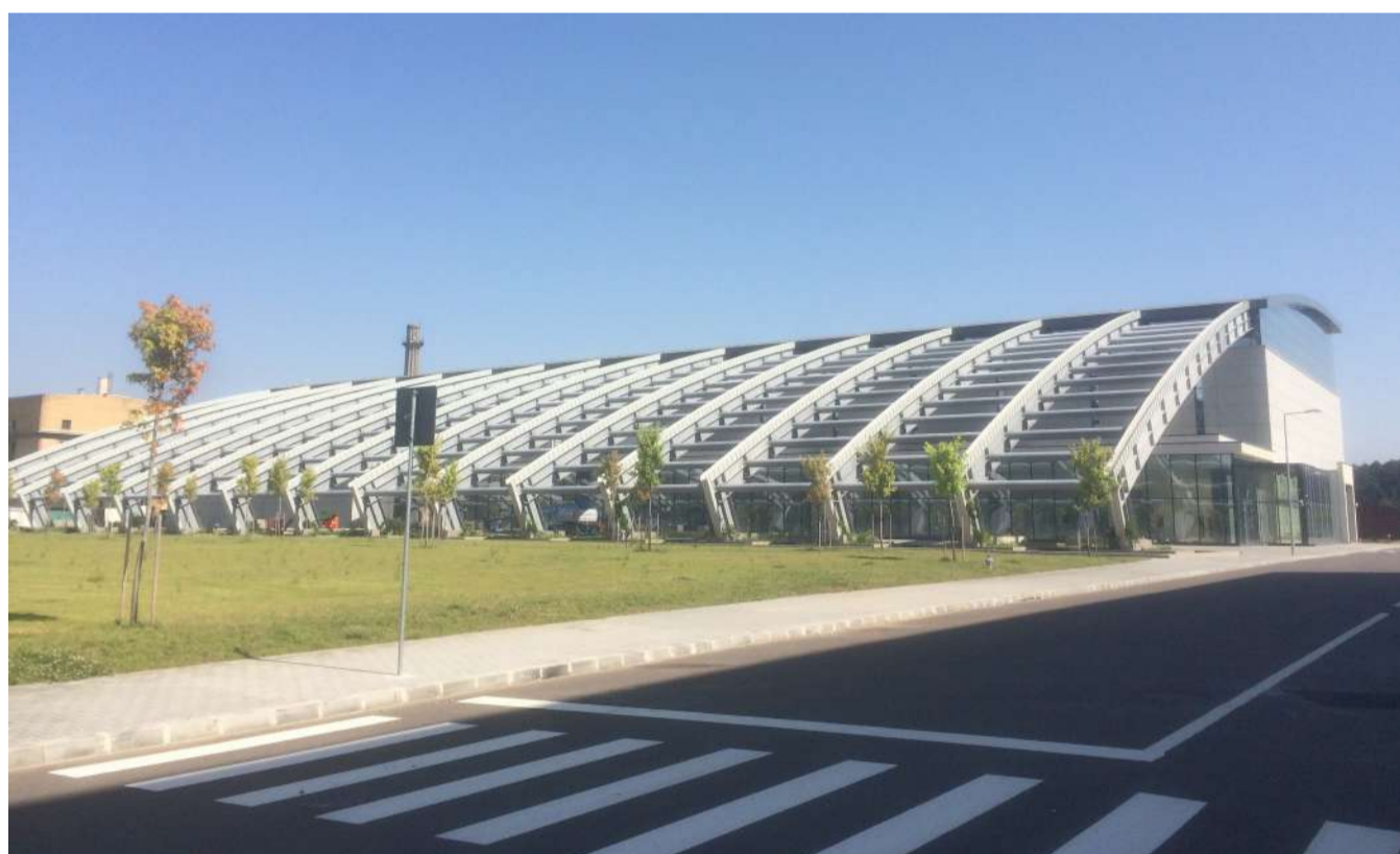
Figure 1: ELI-NP building (Magurele).
